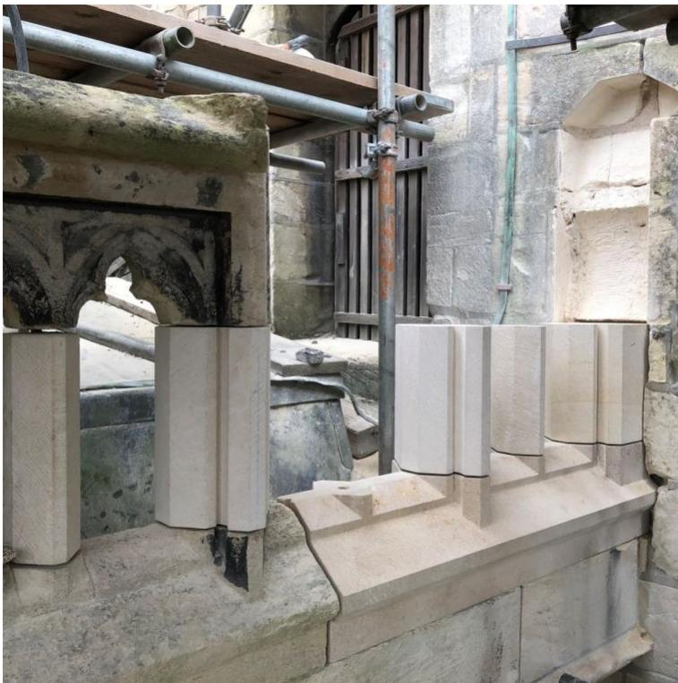
*Figure 4. Cill and mullions, two of which were worked by me, fixed.*
