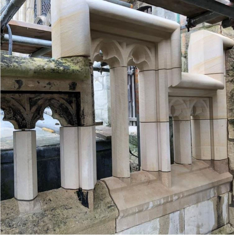
*Figure 5. Full parapet fixed and waiting on final pointing.*
