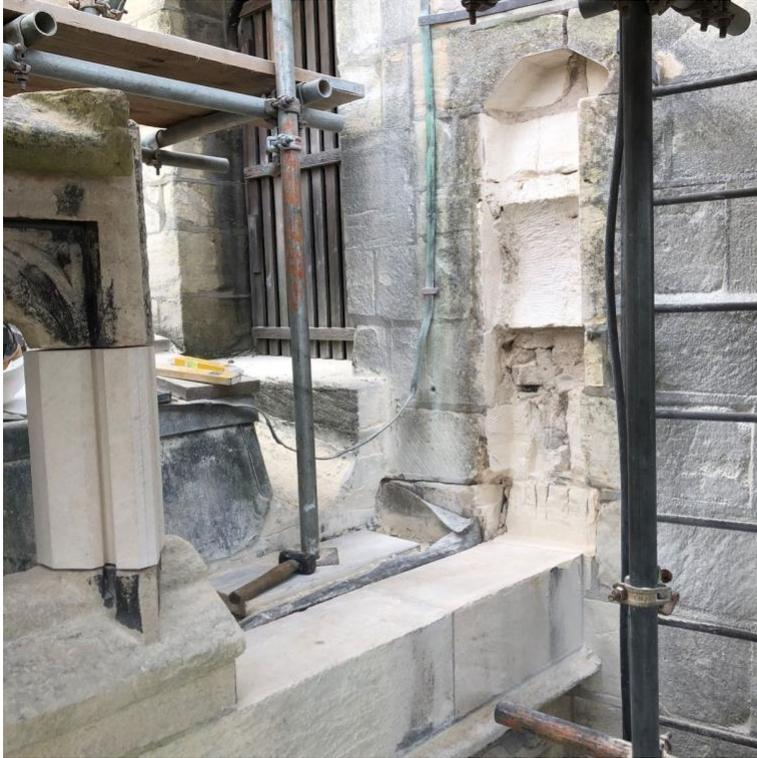
*Figure 3. Original section of parapet dismantled and ready for new masonry*
