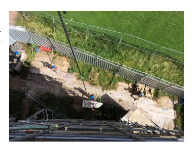
was then laid on a trolley and wheeled into position on the scaffold. Then using a combination of pulley chains and straps, it was slowly and steadily lowered into position. It is quite a sight to behold and a nice process to be a part of.
