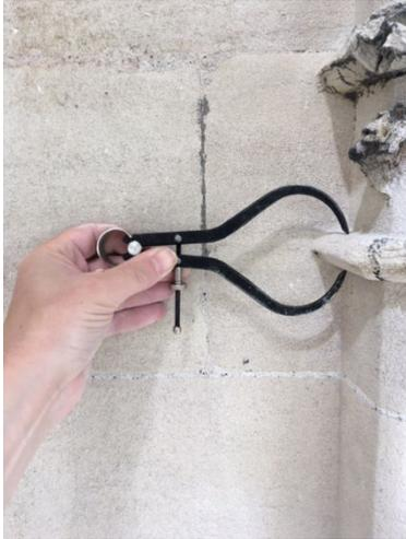
He writes: With my toolkit of dividers, callipers, tape measures, rulers, bevels, a profile gauge, paper and pens I set about taking the various measurements I needed from the capital on the right hand side of the window and from a missing corbel on the left hand side.
