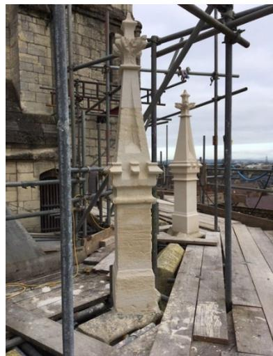
With the poulticing complete, over the past few days I have been cutting out old mortar from the joints of the stones around the window and repointing all of which adds to the longevity of these precious stones.
